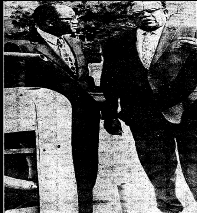
This machine, standing on one of Robbins' few sidewalks, pumps sewage from a low sewer into a higher one. Robbins Mayor Marion Smith (right) explained to Special Presidential Asst. Robert J. Brown that his village has already applied for government help in correcting such problems, but the government has as yet taken no action.
