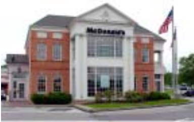
Less architecturally appealing, perhaps, but more context-sensitive is this McDonald's in Independence, Ohio.
