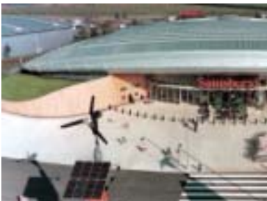
Sainsbury Supermarket, Greenwich, London. 8
