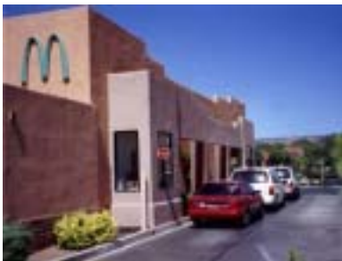
Teal green replaces the golden arches for a Sedona McDonalds; stucco cladding reflects the colors of the Sonoran desert.
