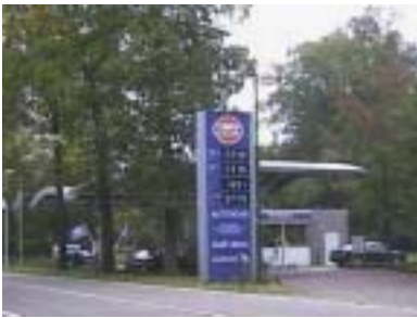
Gulf Station in Bilthoven, the Netherlands, fits into its natural setting. 48
